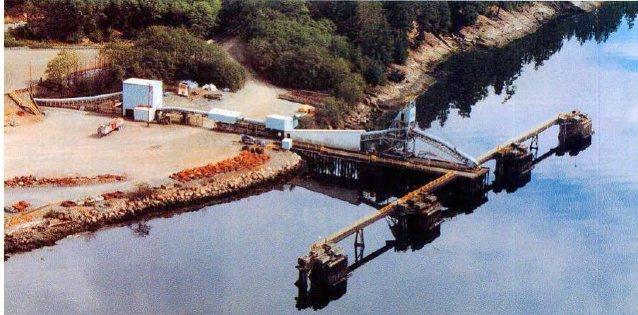
The tidewater loading facilities for BHP Billiton's former Island Copper Mine. Source: Western Copper Corp.
