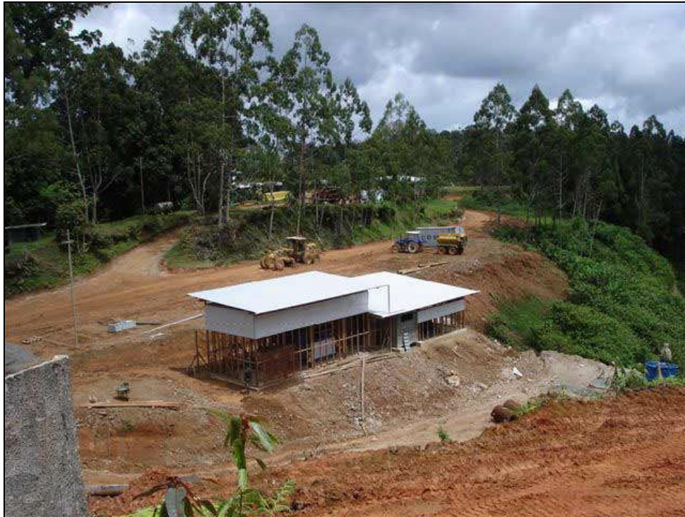
The company's processing plant and laboratory at the Sinivit project.
