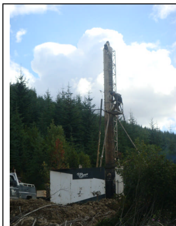
Drilling on the Upper Fir.
